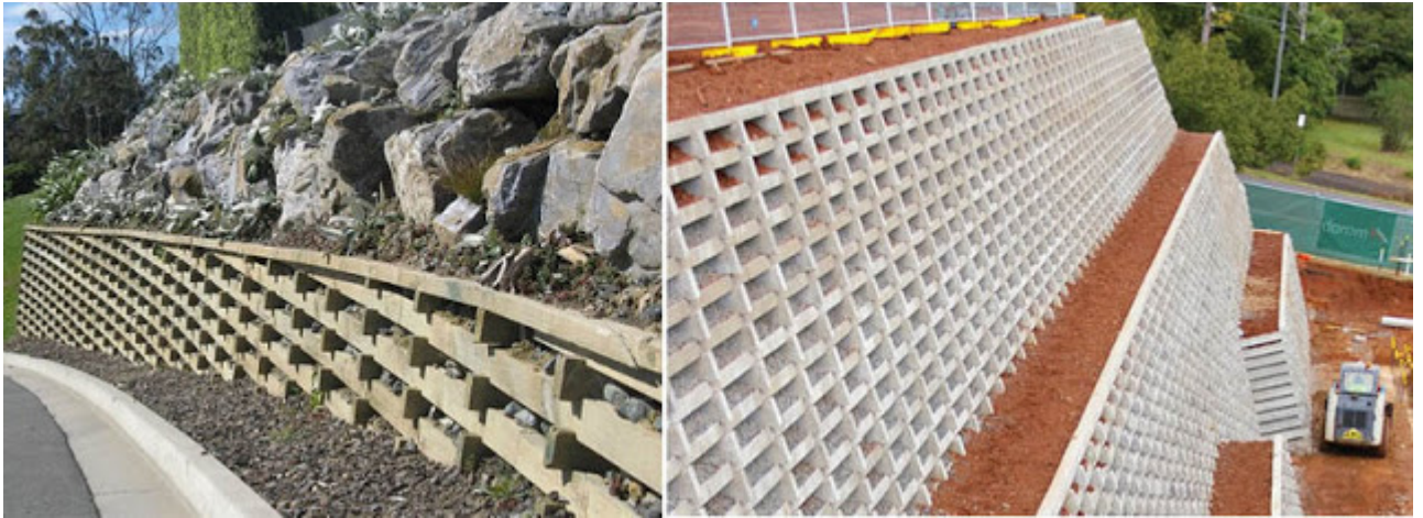
Gambar 11. Struktur Dinding Penahan Reventment
