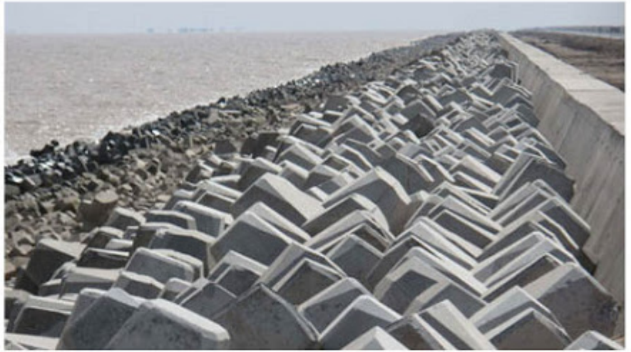
Rubble Concrete Revetment
