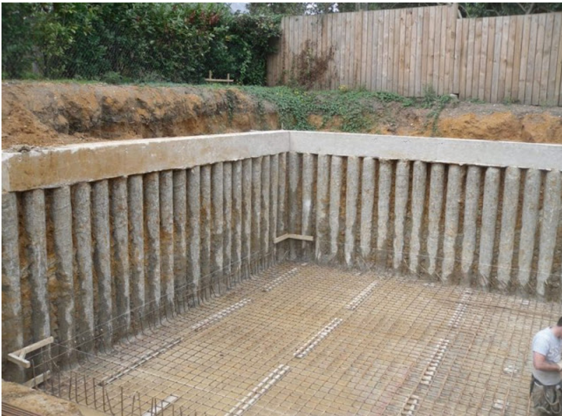
Gambar 9. Struktur Dinding Penahan Tanah Soldier Pile
