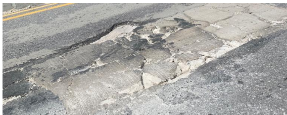
Figure 10 Potholed Road in Rimbo Panjang Village
