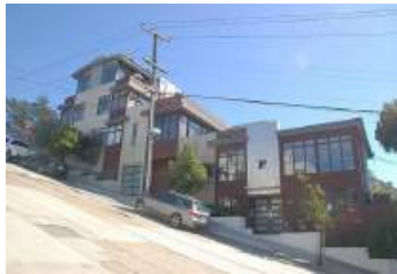
Gambar 3. 18 Ilustrasi sloping site Sumber : (FEMA P-154, 2015)
