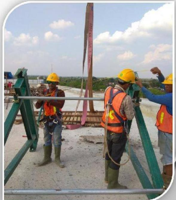
*Gambar 10. Pemasangan Climbing Bracket*
