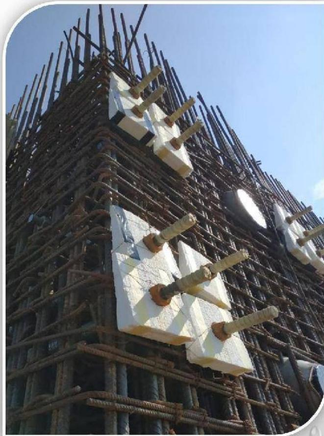
*Gambar 35. Post Tension Bar terpasang*
