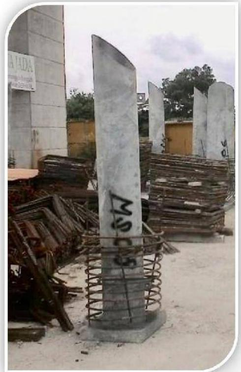
Gambar 32. Bursting steel guide pipe
