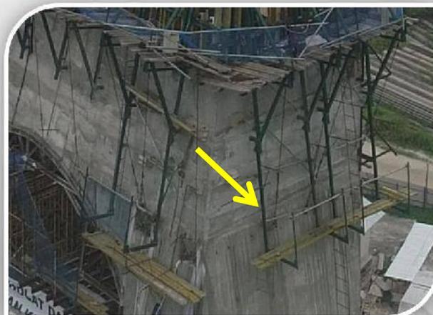
Gambar 16. *Suspended Platform* terpasang
