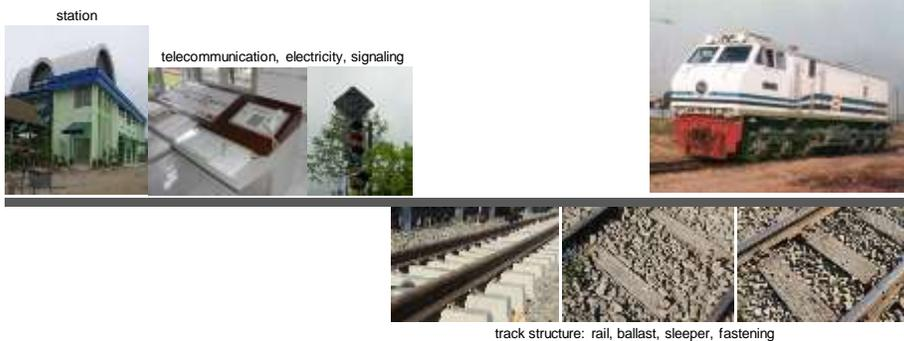
track structure: rail, ballast, sleeper, fastening
